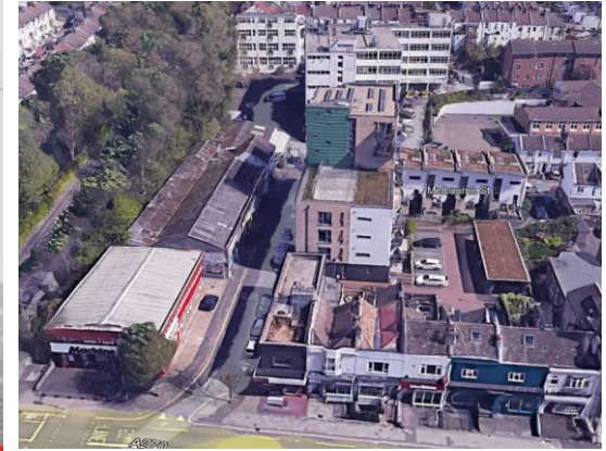
Existing Viaduct Lofts
